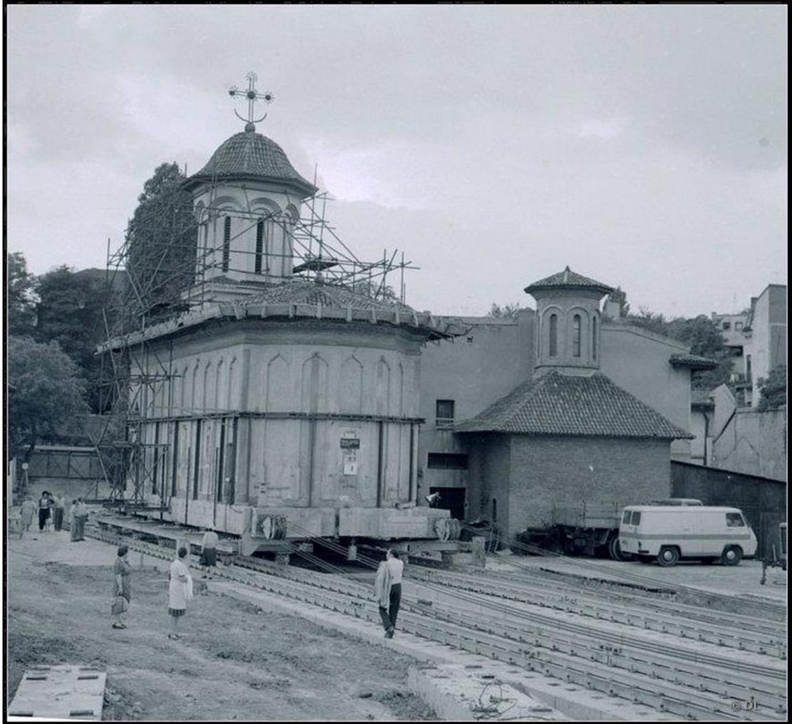
Image 33 - The small church is being moved to the new site, 200 meters away, documentation photograph. Source: [www.rezistent.net](http://www.rezistent.net).
